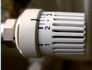
But the thermostat valve can only work properly if it is not blocked by furniture or curtains.
