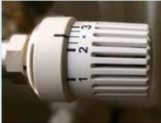
But the thermostat valve can only work properly if it is not blocked by furniture or curtains.
